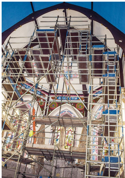
Left: Example of the extensive scaffolding required for the decoration
